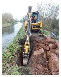
Whilst there at that location the opportunity was taken to widen the approaches to Ayshford Bridge, which were narrow and uneven. This was done by scraping out the path and then resurfacing with a few tonnes of limestone scalpings.
